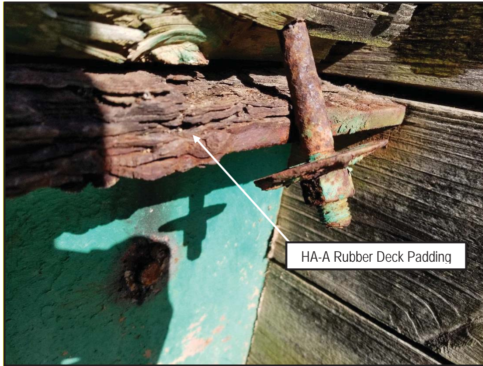
Photo 1: View of HA-A on the SR-87 bridge over Overflow
