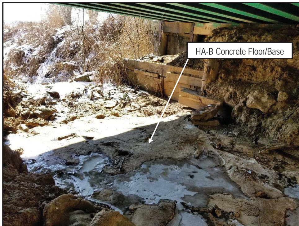
Photo 2: View of HA-B on the SR-87 bridge over Overflow
